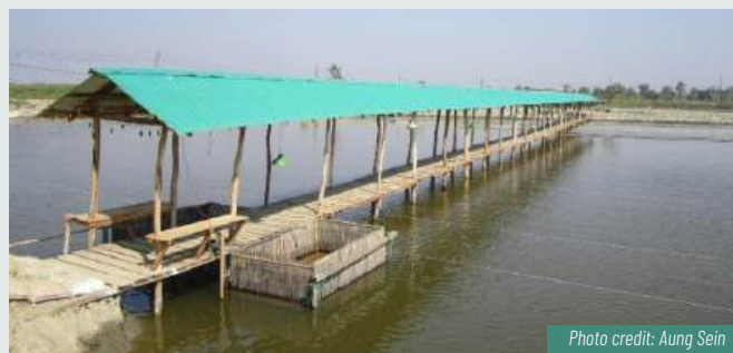
Shaded pontoon bridge.
